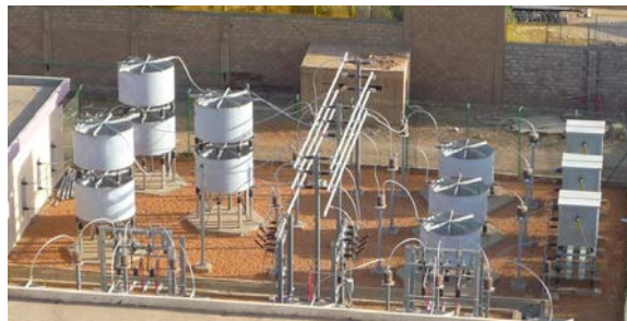
Fig. 1: Static var compensator at steel mill (MP, 2018)
