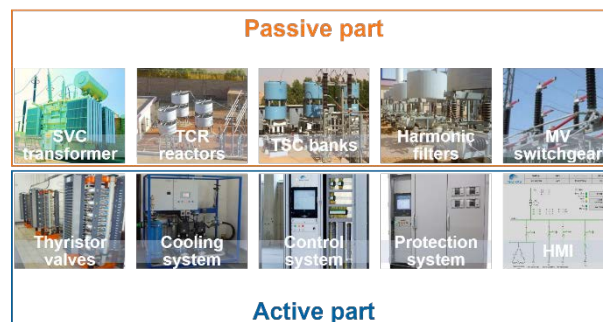
Fig. 4: Main components of an SVC
