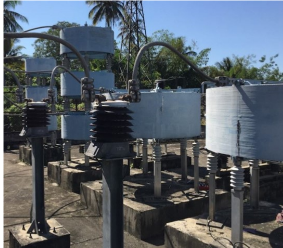
Fig. 12: Harmonic filters and TCR reactors (MP, 2018)
