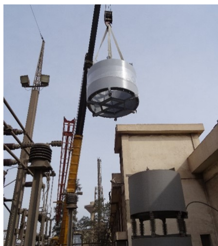
Fig. 13: Installation of TCR reactors (MP, 2018)
